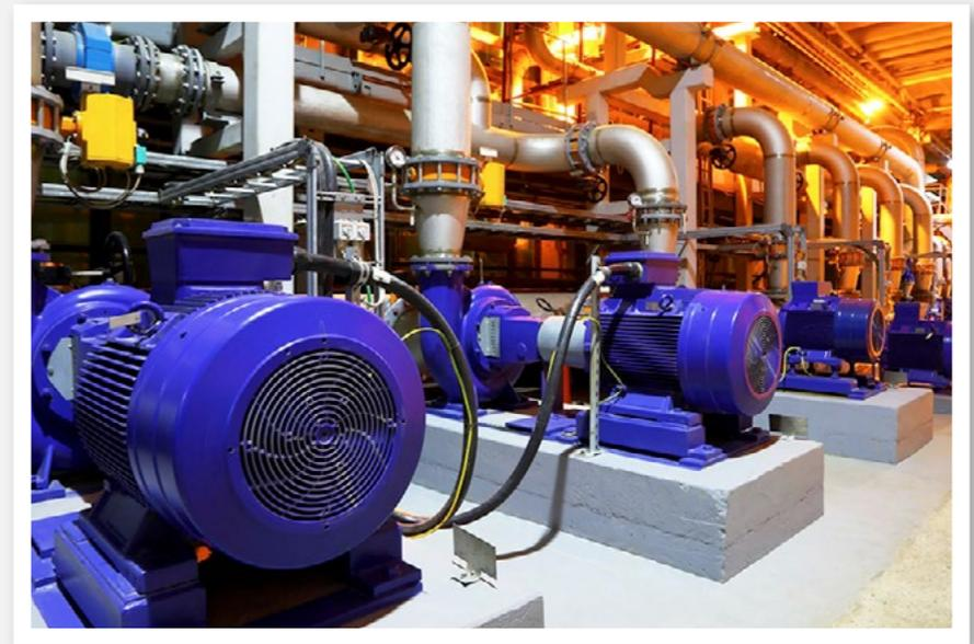
**Energy-efficient electric motors** The largest energy consumers in industry are electric motors: they account for around two thirds of total electricity consumption. An analysis by Bilfinger Chemserv at an industrial park in Linz came to the conclusion that, of the 3,000 motors in use there, around 1,000 needed to be replaced. The potential energy savings were quantified at a yearly 6,200 MWh, or €370,000 per year. The investment will pay for itself within two years.
