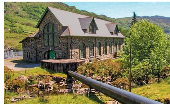
The landmark-status Cwm Dyli hydro power plant in the Welsh region of Snowdonia went into operation in 1906. It feeds around ten megawatts of electricity into the grid. The water that turns the turbine comes from the Llyn Llydaw lake, 320 meters above the plant. Bilfinger UK has now been awarded the contract by the operator Innogy to refurbish the plant's instrumentation and control technology.
