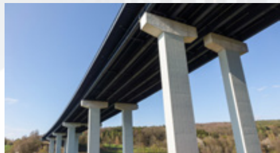
Alluring, but ailing: The Thalaubach viaduct in Germany's federal state of Hesse is to be replaced with a new structure starting in 2022.
