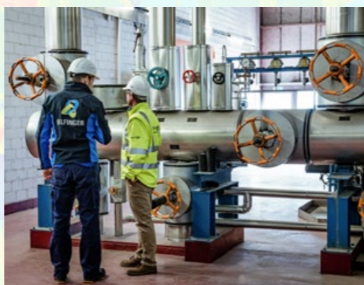
Searching for lost heat: Specialists at a wood-fired heating plant in Canton Uri.
