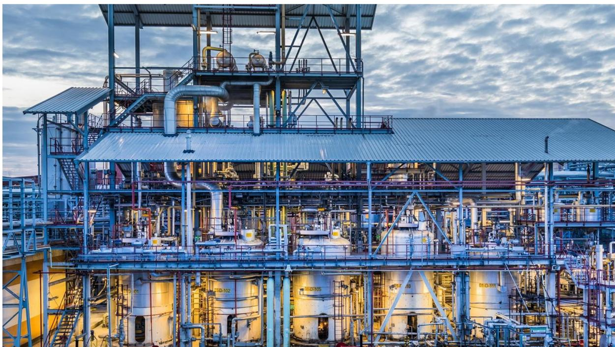
Capture: One source of hydrogen is from the chloralkali electrolysis in the production of chlorine. The hydrogen by-product can then be, cleaned, cooled and compressed for onwards transportation by road, rail or pipeline. Copyright: Spolchemie
