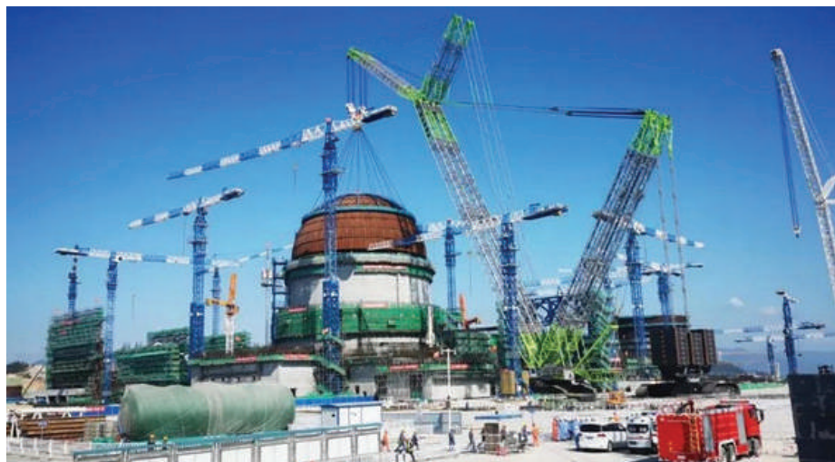
LIFT The inner dome of the Zhangzhou nuclear power plant's first unit is installed in China's Fujian province. Units 1 and 2 are set to operate in 2024 and 2025, respectively.
