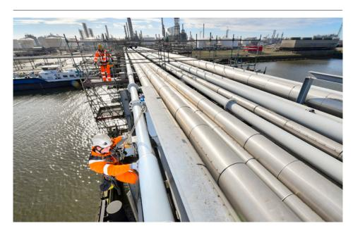
Shell Moerdijk called on Bilfinger's new expertise for the rapid and efficient inspection of its T-jetty – and also benefited from significant financial savings. This inspection work is part of a special Shell programme focused on the prevention of corrosion. The use of rope access together with supplementary inspection expertise yielded considerable benefits.
