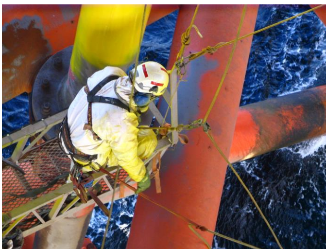
Bilfinger E&M UK will carry out operations and maintenance services for the floating offshore wind farms
