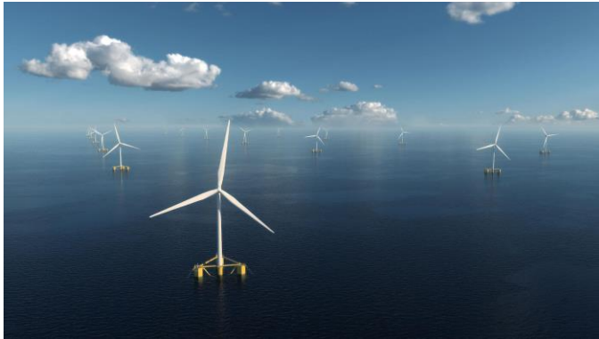
Floating offshore wind turbine foundations. © Cerulean Winds
