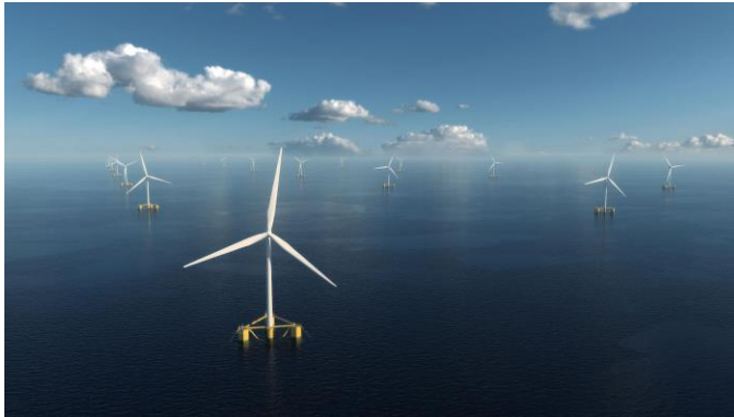
Floating-Offshore-Windturbinen. © Cerulean Winds
