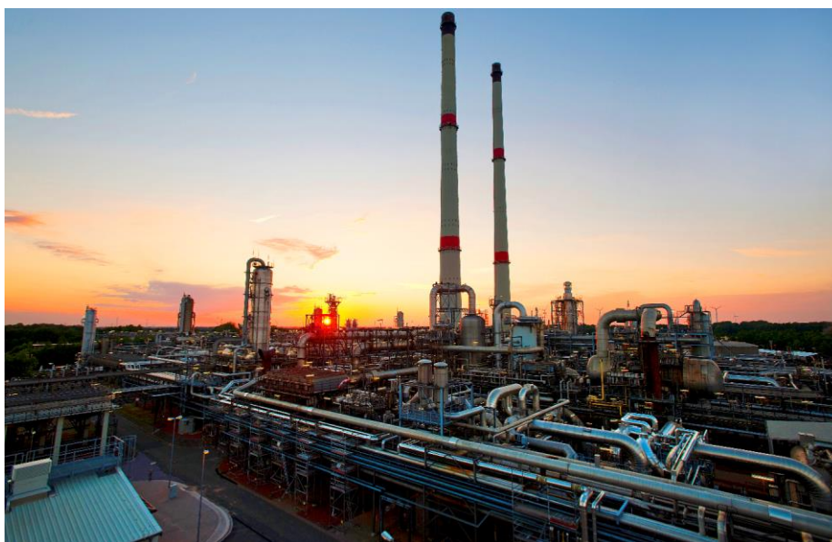
ExxonMobil natural gas processing plant in Großenkneten © ExxonMobil
