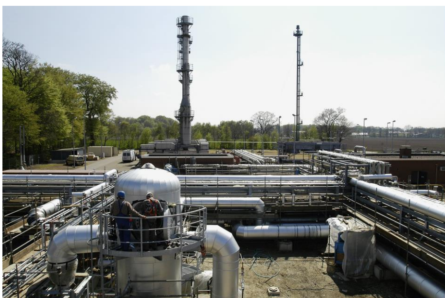
Work on the Visbek compressor station in southern Oldenburg © ExxonMobil
