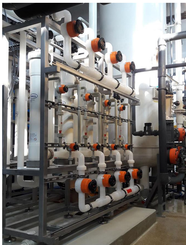
Filtration unit for ultra-pure water with high-purity PVDF material
