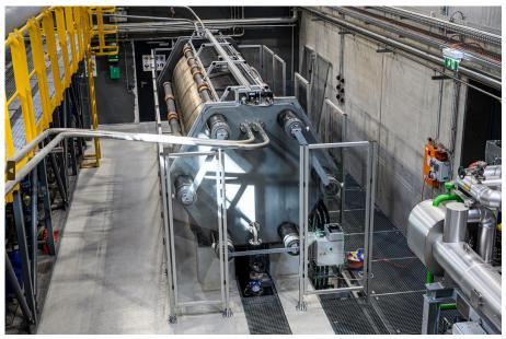
Europe's largest single-stack electrolysis plant, which produces green hydrogen using green electricity at the MPreis site in Völs near the Austrian city of Innsbruck. © MPREIS / Franz Oss
