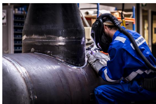
Prefab work by De Bruin specialists
