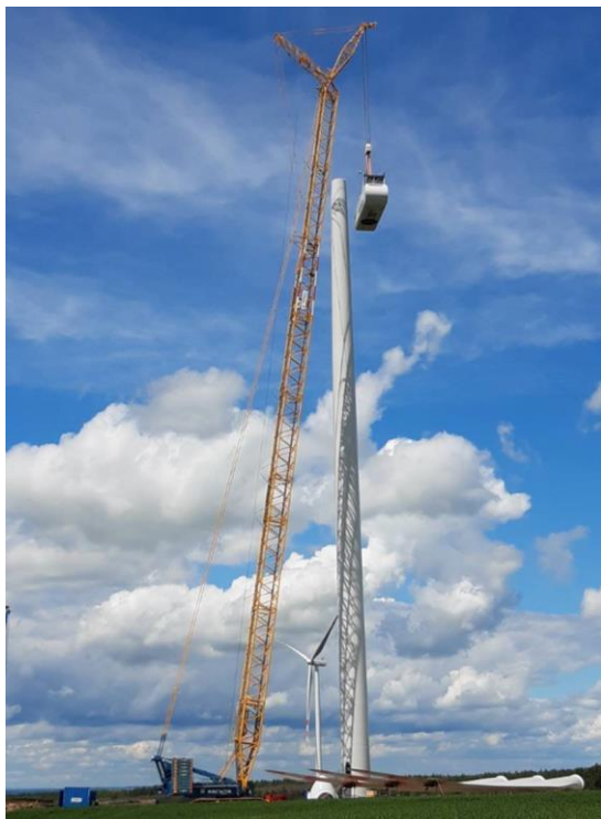
Construction of the EDF Górzycza wind farm
