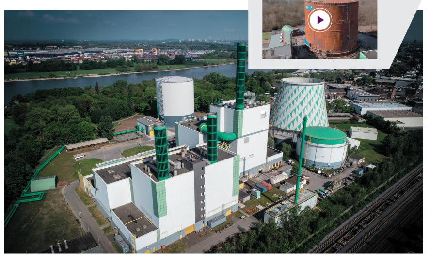
A Bilfinger two-zone district heating accumulator increases the efficiency of the Duisburg public utility company's thermal power station.
