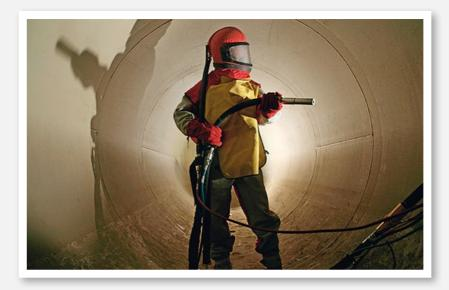
Bilfinger Grit Ann Coyne and Simon Hope of Bilfinger Salamis have developed a particularly environmentally-friendly material for surface blasting. "Bilfinger Grit" is a blend of recycled glass and blast furnace slag. It is now increasingly used at Bilfinger in place of the usual garnet sand to clean steel structures prior to re-coating. Demand is several thousand tons per year.
