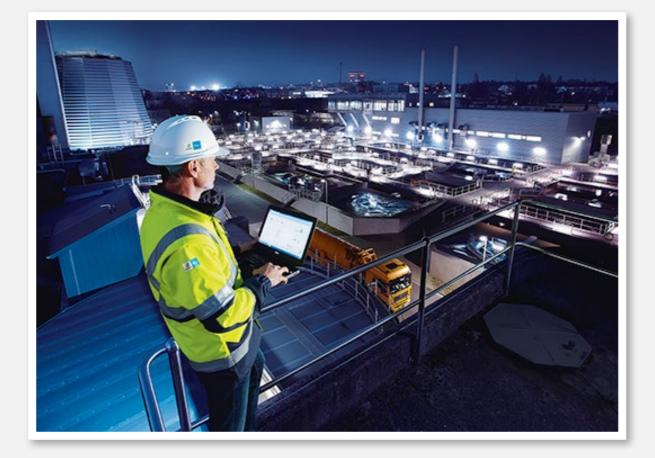
**Millions of little helpers** In the main sewage treatment plant in Wiesbaden, countless microorganisms purify around 50,000 cubic meters of wastewater each day. In recent years, Bilfinger Water Technologies has planned and realized various processing steps for the treatment plant, from fine screening and biological treatment to secondary clarification.
