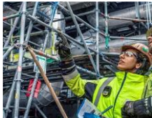
Insulation, Scaffolding & Painting
