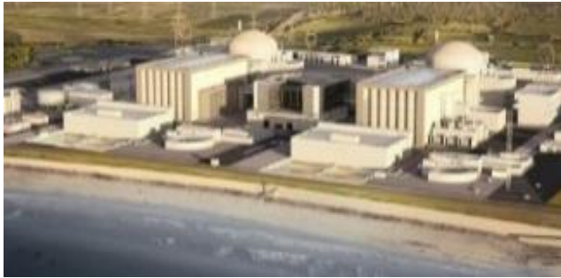
EDF Hinkley Point United Kingdom
