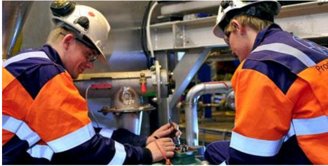
MAINTENANCE SERVICES (BMC)
