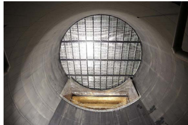
Interior view Tray Absorber
