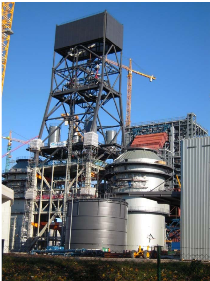
FGD Moorburg Power Plant
