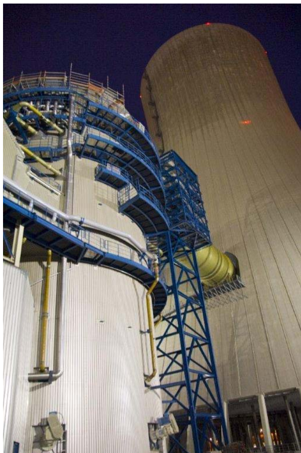
FGD Boxberg Power Plant
