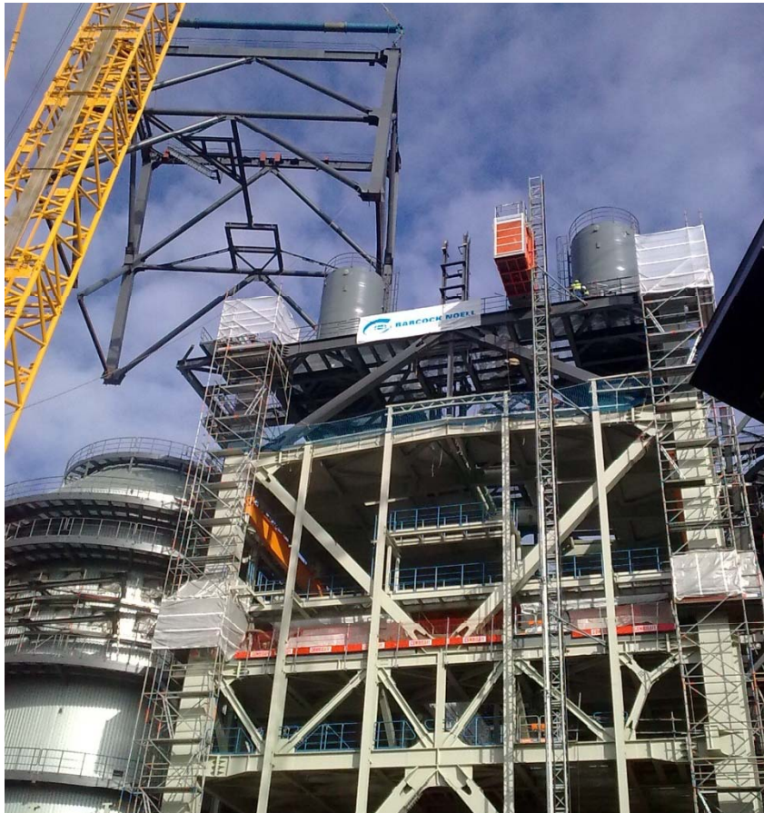
FGD Moorburg Power Plant
