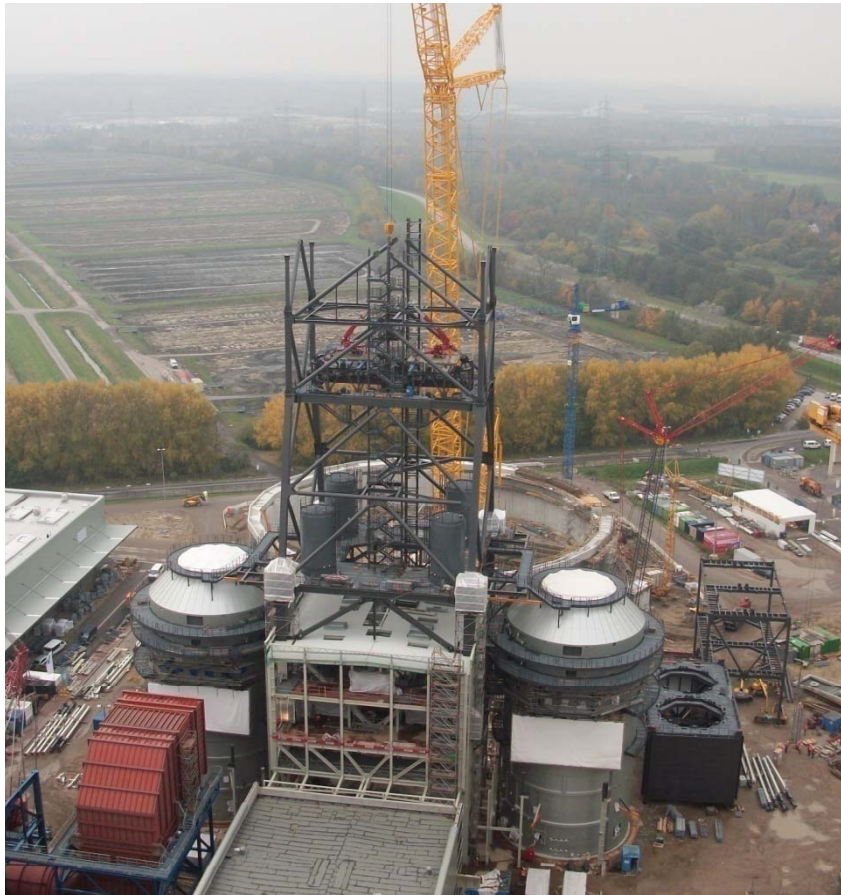
FGD Moorburg Power Plant
