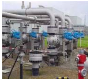
Valves Flow Measurements
