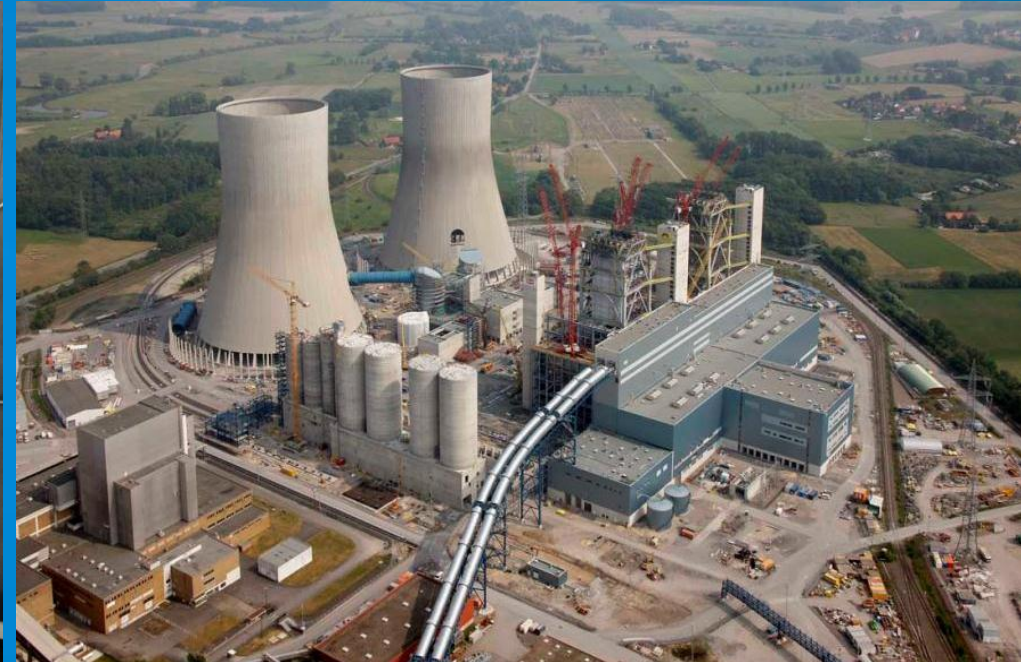
Bilfinger Envi Con | Engineering Power Plant Westfalen / RWE, Block D & E | Germany
