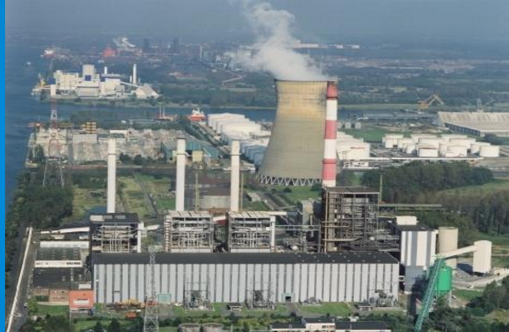
Babcock Borsig Steinmüller | Upgrading and efficiency improvement Rodenhuize power plant | Belgium
