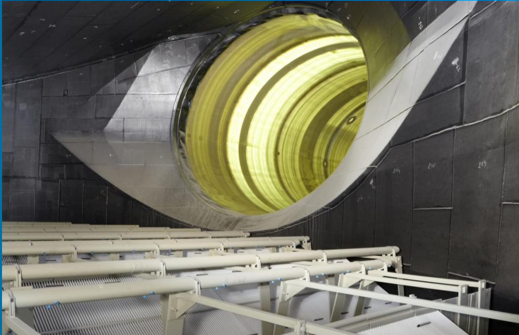
Babcock Noell | Heat recovery from flue gas Boxberg power plant | Germany
