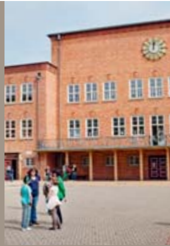
The Pestalozzi School building, built in 1929, was modernized by Bilfinger.
