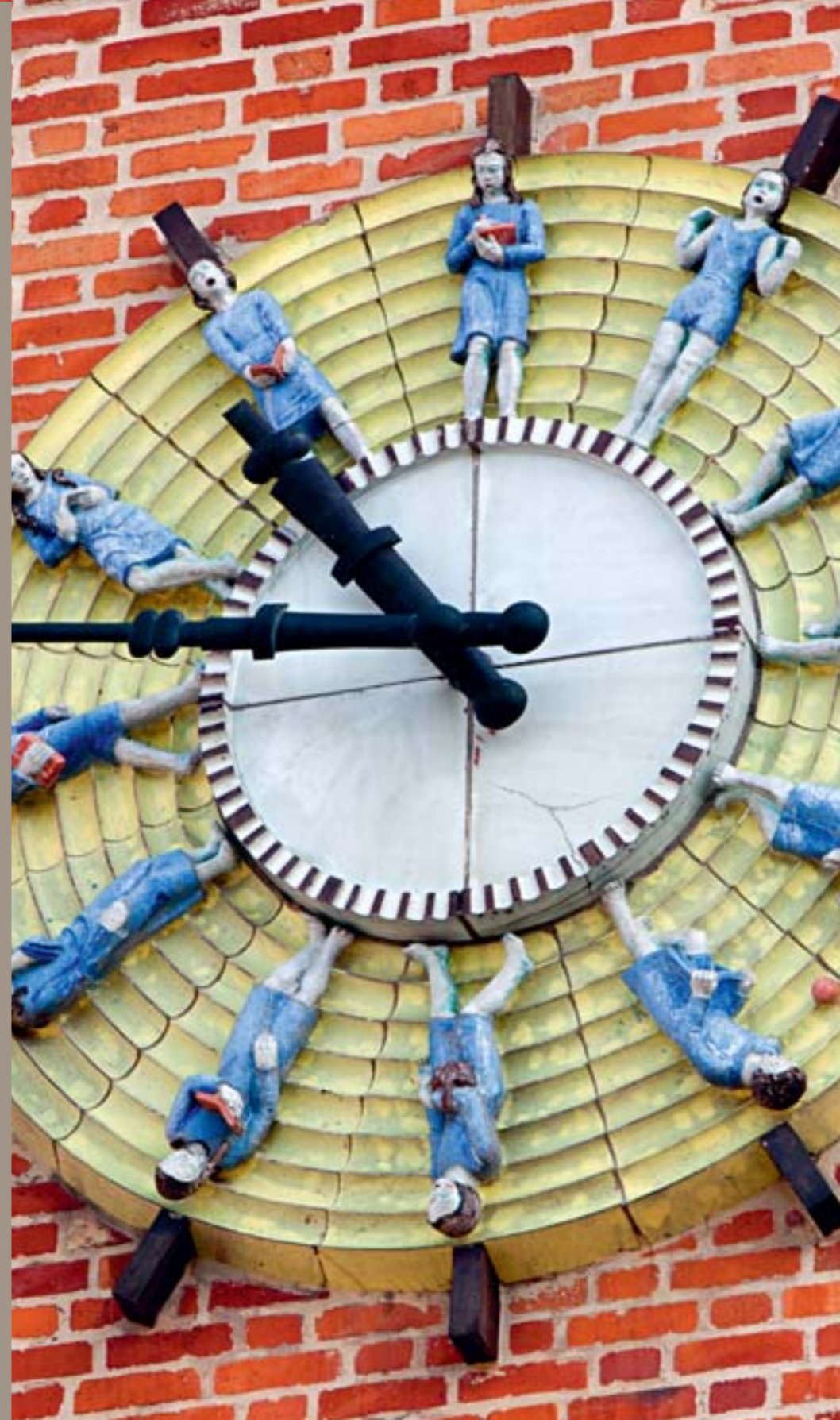
11 o'clock: singing, 12 o'clock: writing, 1 o'clock: gym. The old school clock shows diligent students and their daily routine. The clock hadn't worked since the 1980s. Bilfinger restored it in collaboration with a local clockmaker.
